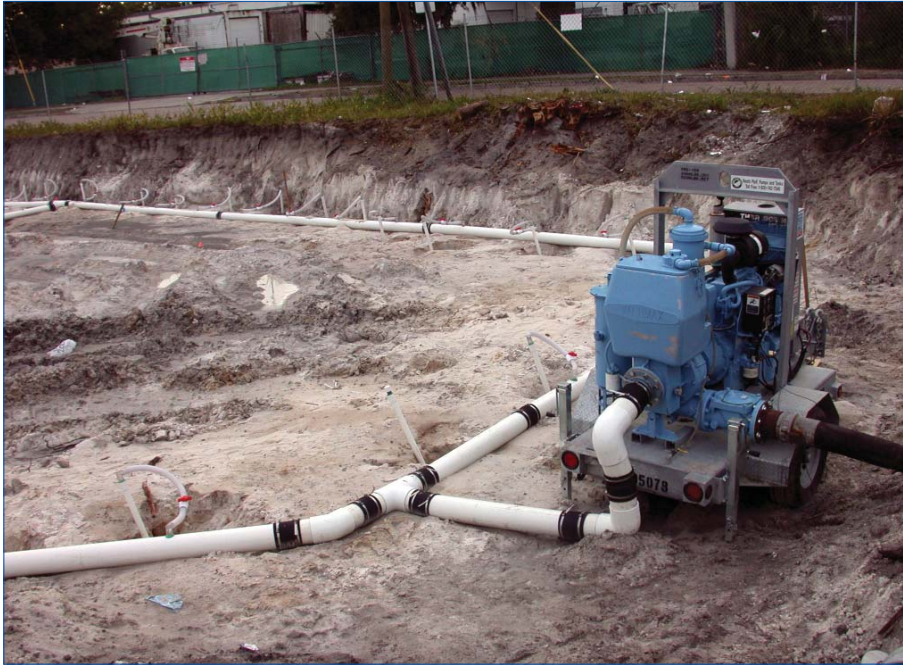
The main types of pumps used in wellpoint dewatering are centrifugal pumps, which come with a variety of features and capabilities to suit different needs.
