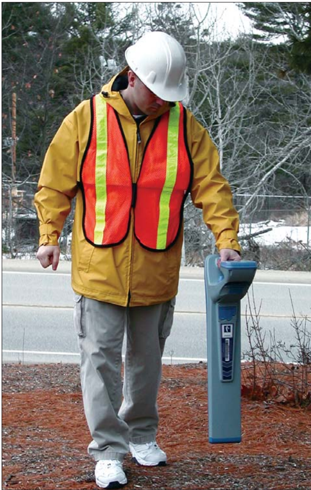
Visual confirmation is advocated by locator manufacturers across the board, because while locators can get you very close, they aren't 100 percent accurate either.
